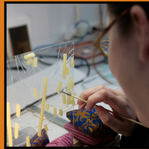
Application of adhesive to vertically assembled, non-planar window glass photograph by Ralph Wiegandt
